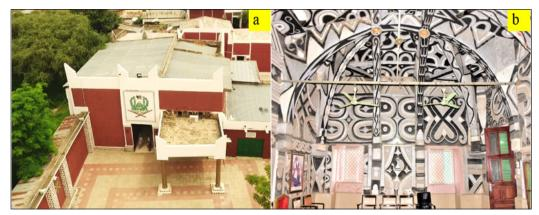
Figure 7. (a) Aerial view of the monumental guest-chamber Soron Giwa, showing the zinc roof sealing the mud roof and then cladded with the masonry wall; (b) The preserved interior of soron Giwa in its earthen form
